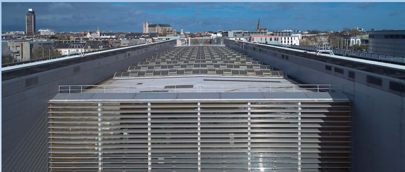
ARMOR's OPV (Organic Photovoltaic) film solution has been applied to the Cité des Congrès building in Nantes, France. (Photo credit: G. Satre.)
